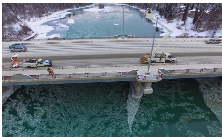
Soldotna Bridge Photo by: Jeff Jicha
