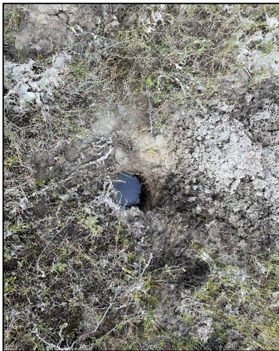
Photograph 4: Groundwater immediately below ground surface.
