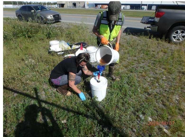
IDW decon water treatment using a 5-gallon GAC and onsite disposal
