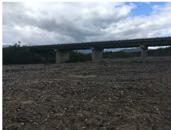
Figure 40. Dry Creek Bridge (BR 0851), Downstream Looking Upstream and South
