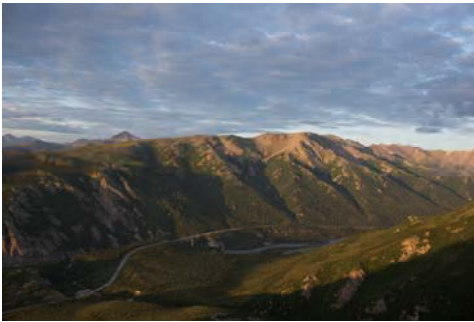
Roadway geometry (~MP 243.5)
