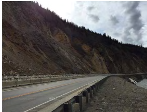
Nenana Canyon rockfall area (~MP 240)
