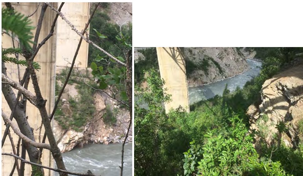
Figure 34. Looking Downstream, Left Pier and Right Abutment
