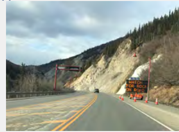
Rockfall hazards (MP 239-241)
