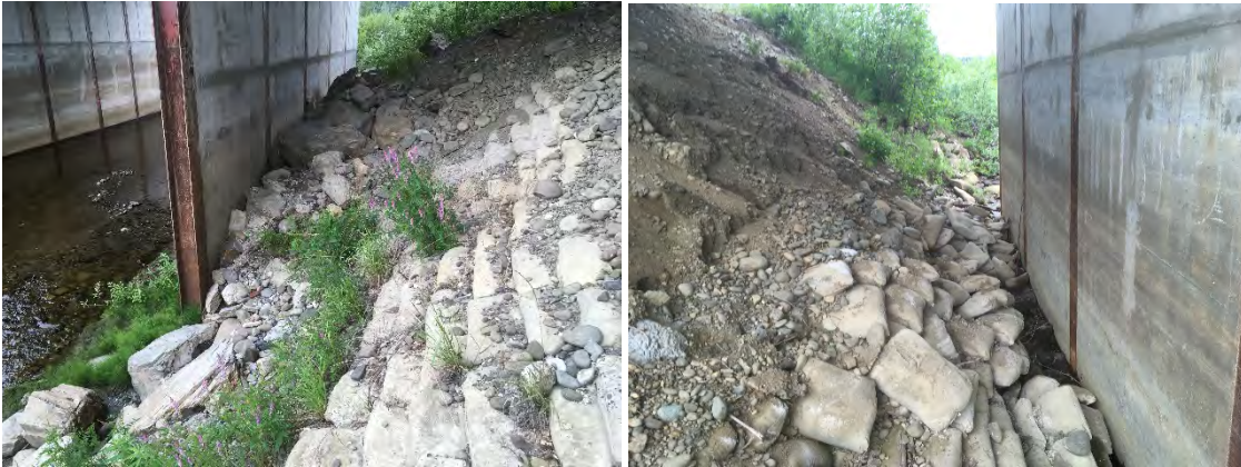
Figure 43. Looking Upstream, Left Abutment: Looking Downstream, Right Abutment
