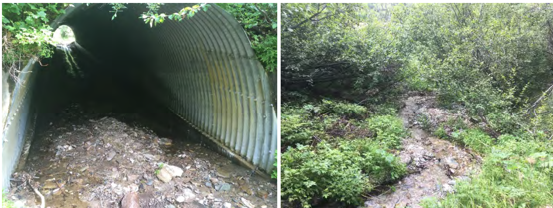
Figure 29. From Downstream Side Looking Upstream and Downstream
