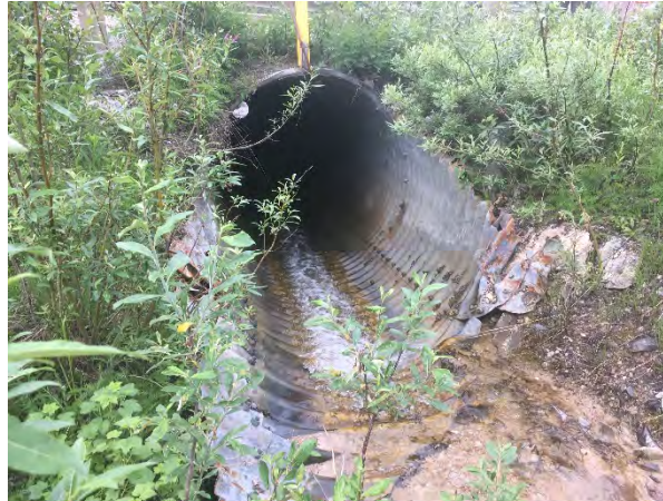
Figure 20. Junco Creek Cross Culvert, Upstream Looking Downstream
