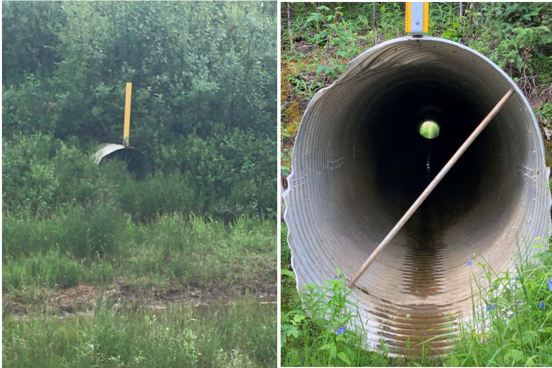
Figure 60. Culvert at MP 248.4: From Upstream Looking Downstream: From Downstream Looking Upstream
