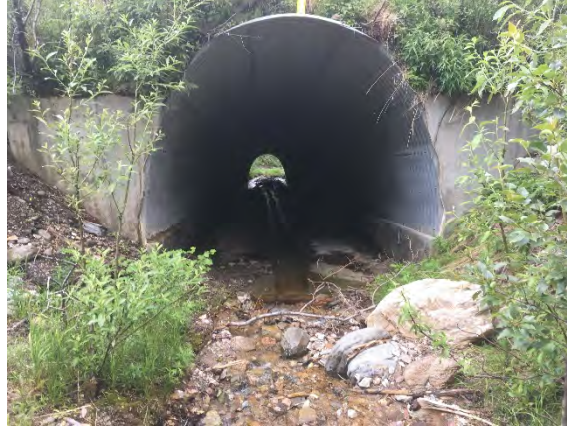
Figure 28. Eagle Creek Cross Culvert (7111/1076), Upstream Looking Downstream
