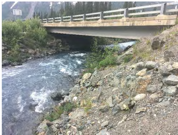
Figure 10. Carlo Creek Bridge (BR 0693), Upstream Looking Downstream
