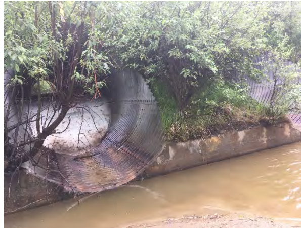
Figure 45. Slate Creek Cross Culverts, Downstream Side Looking Upstream
