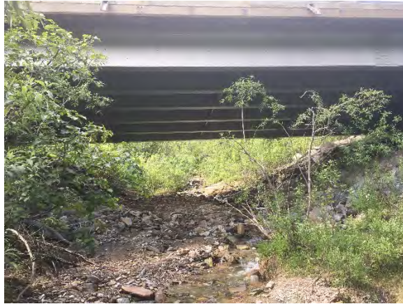
Figure 30. Dragonfly Creek Bridge (BR 1075), Downstream Looking Upstream
