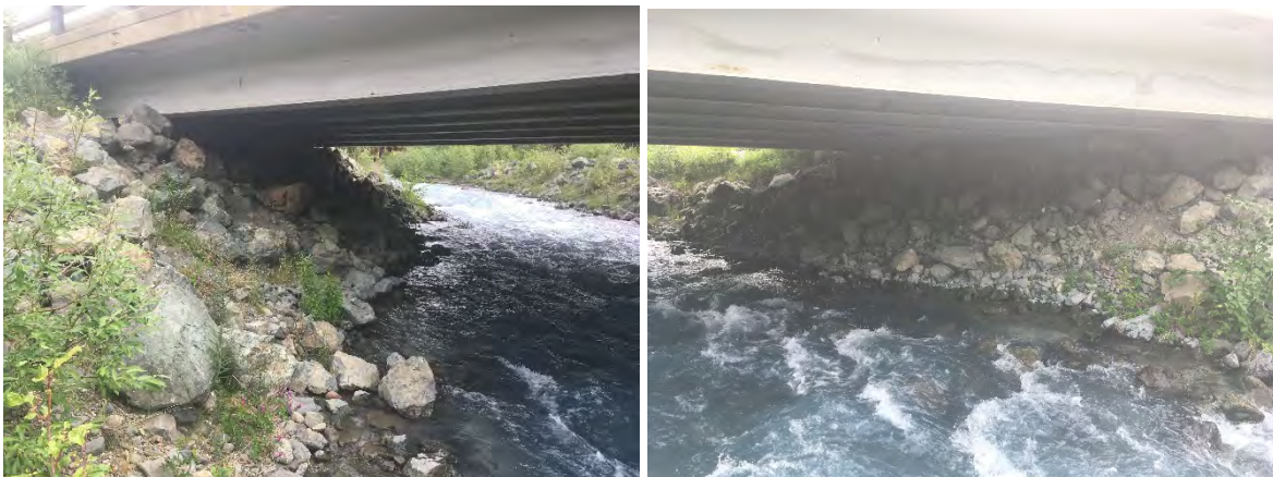
Figure 11. Looking Upstream, Left and Right Abutment
