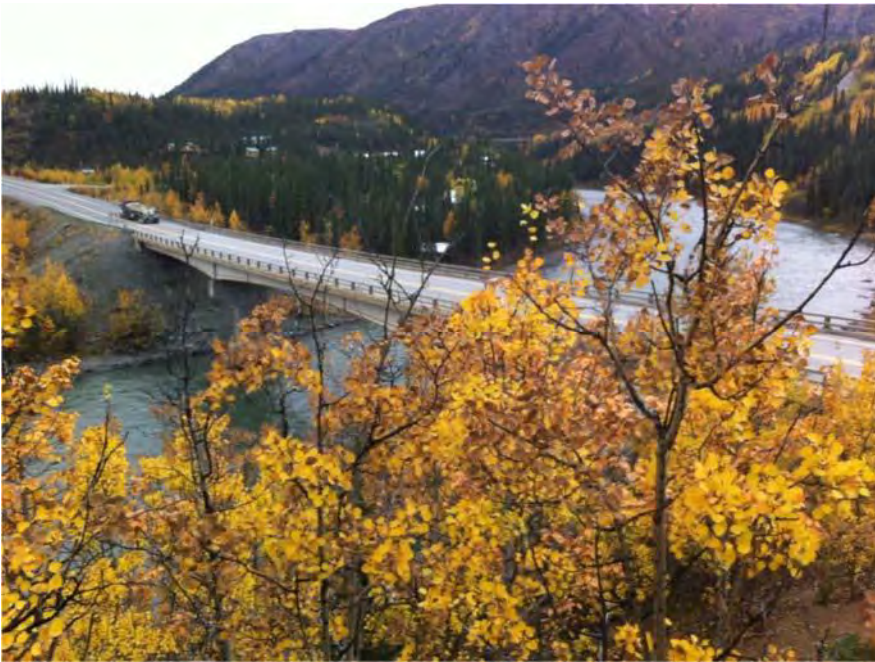
Existing bridge over Nenana River (#694)
