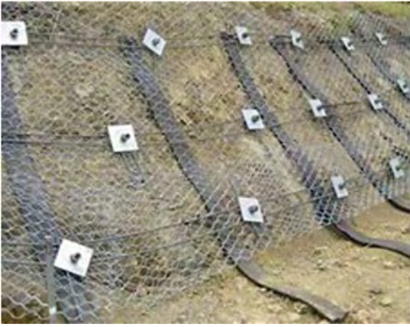
Nenana Canyon rockfall mitigation – rock bolting & netting techniques
