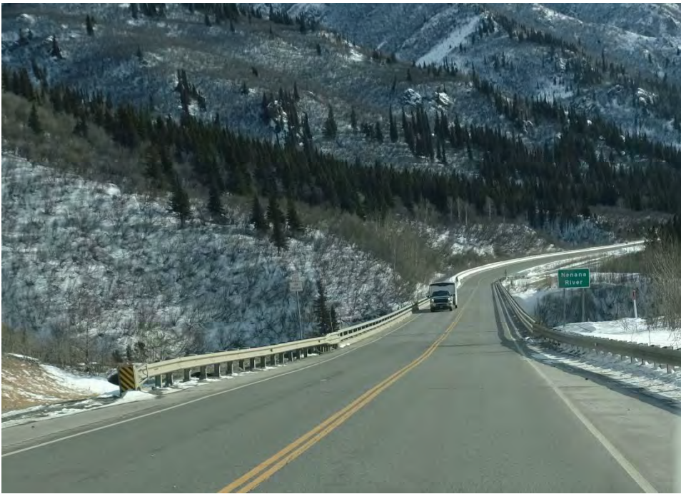
Nenana River bridge, located north of Nenana Canyon near MP 243, is one of several “pinch points” in the corridor for pedestrians: the highway shoulders are narrow.
