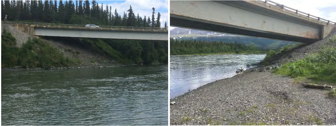
Figure 7. Looking Upstream, Left and Right Abutment
