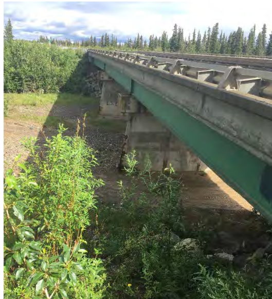
Figure 38. Dry Creek Overflow Bridge (BR 0852), Downstream Looking Upstream and Northwest
