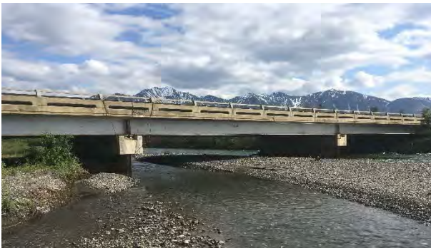
Jack River Bridge, downstream looking upstream
