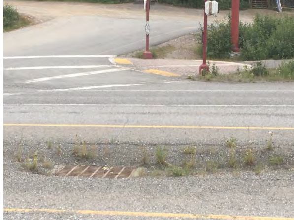
Figure 56. Storm Drain Median Inlet Near MP 238.6
