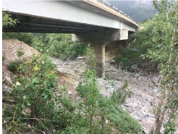
Figure 35. Bison Gulch Bridge (BR 1142), Downstream Looking Upstream and East
