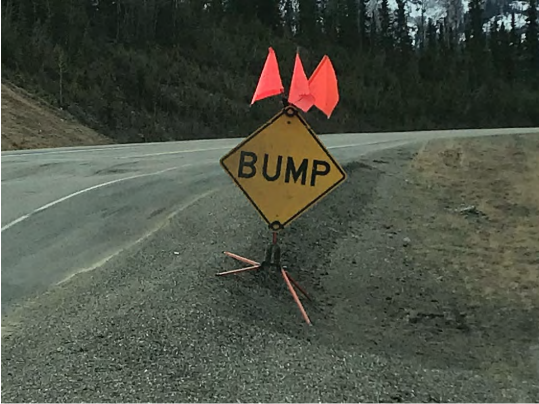
Figure 7 - Additional photo of bumpy section near MP 232.5
