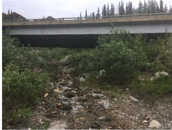
Figure 18. Kingfisher Creek Bridge (BR 0697), Downstream Looking Upstream
