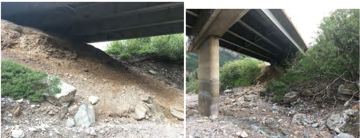
Figure 36. Looking Downstream, Left and Right Abutment
