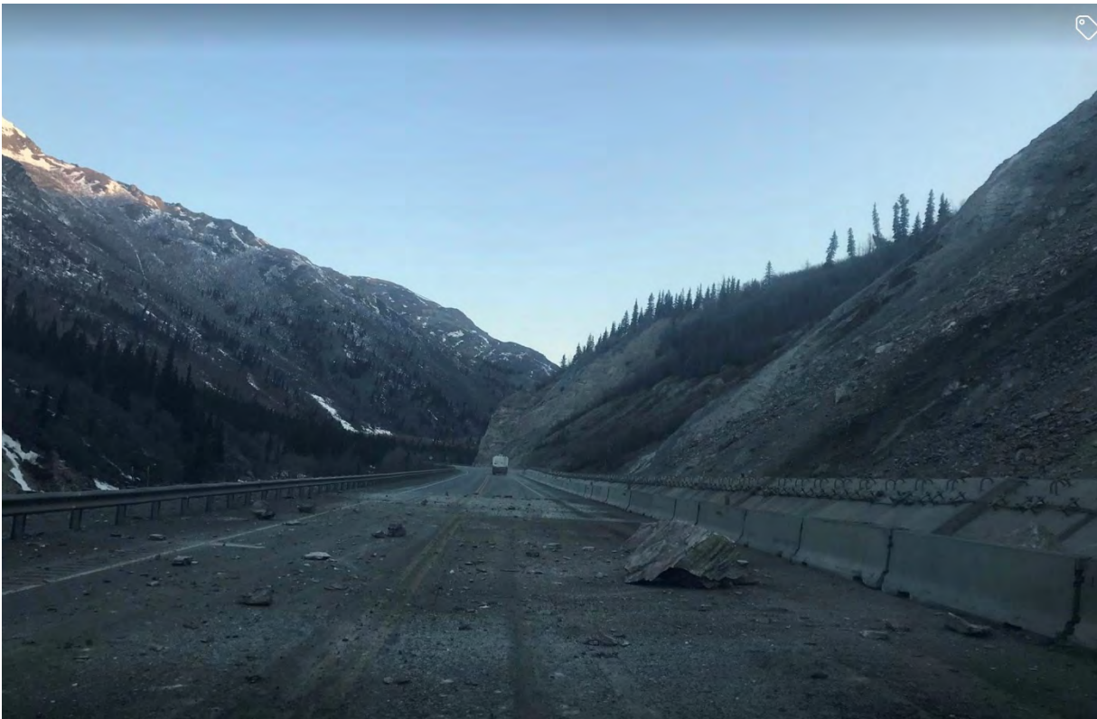
Figure 17 – Larger rockslide that has traveled onto the Parks Highway in Nenana Canyon
