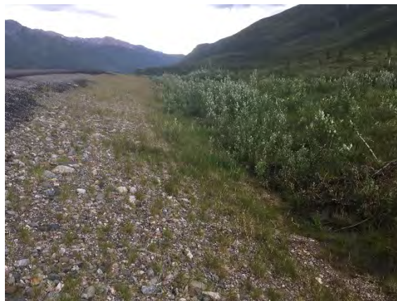
Figure 59. Roadside Ditch Low Point on the West Side Near MP 244
