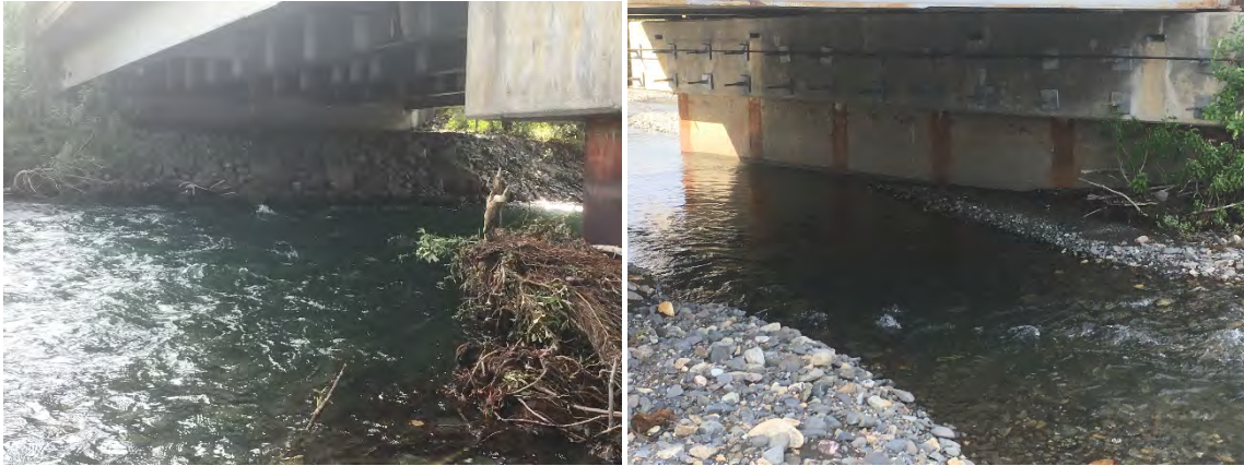
Figure 5. Looking Downstream, Left Abutment: Looking Upstream, Right Pier
