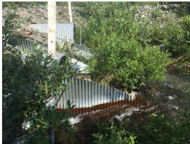
Figure 8. Slime Creek Cross Culverts, Upstream Side Looking North
