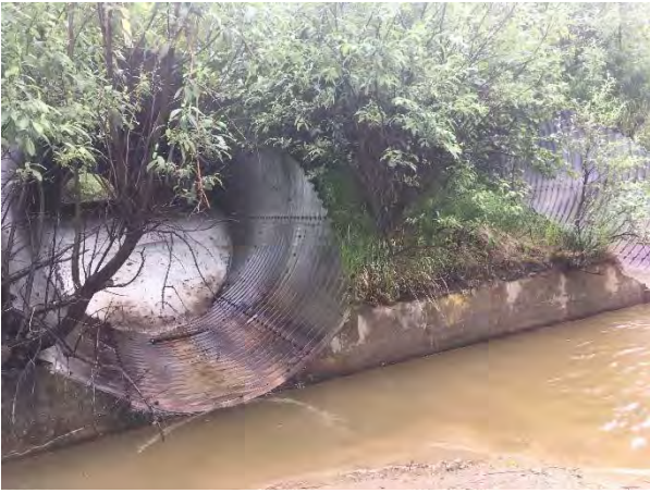
Slate Creek cross culverts (near MP 257.8)
