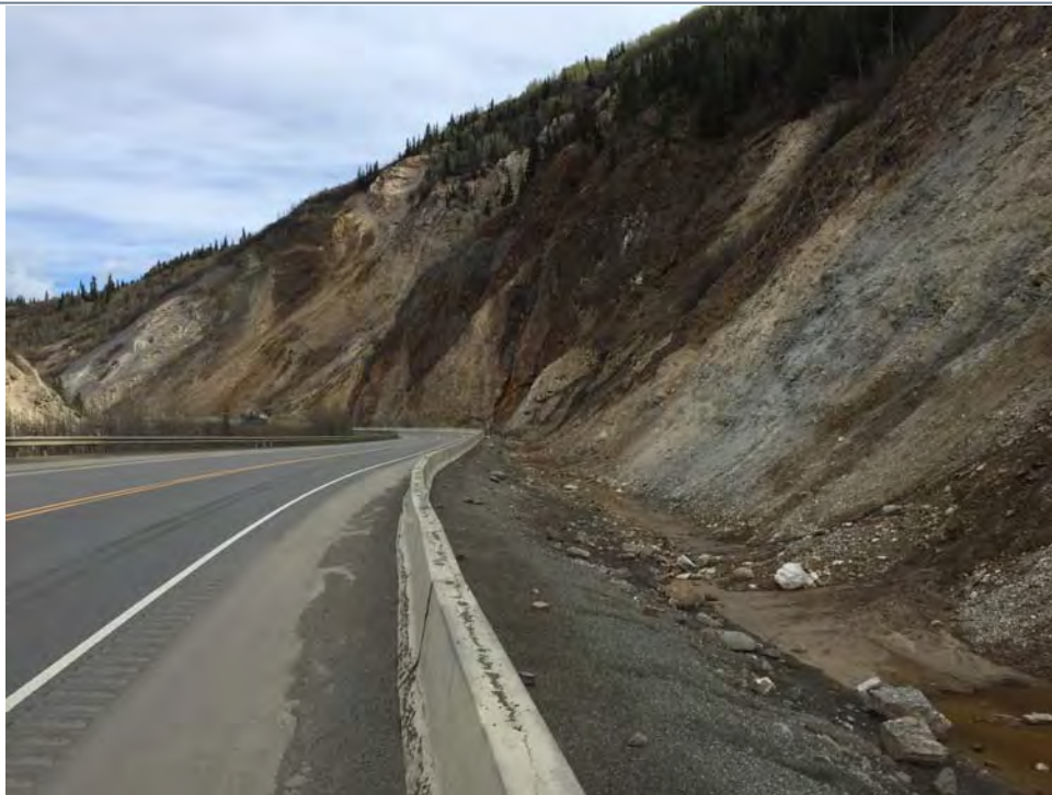
Photo 18: MP 239.2 Widened ditch with concrete traffic barrier. Some rockfall debris in ditch.
