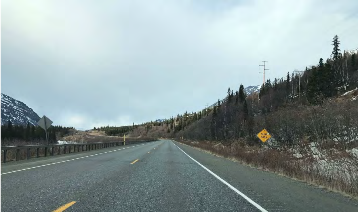
Slide area north of MP 219
