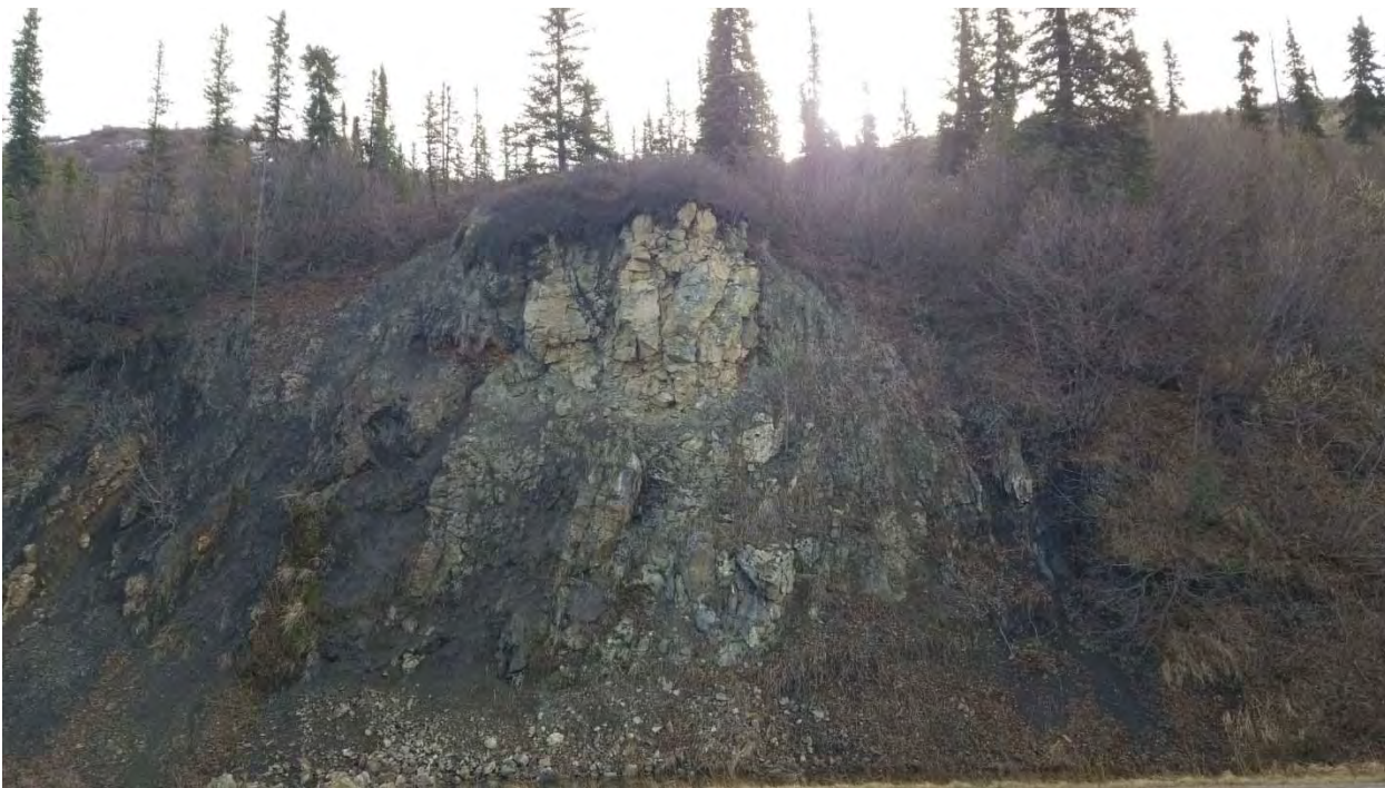
Rockfall near MP 212
