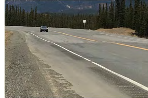
Annual pavement maintenance (~MP 232.7)
