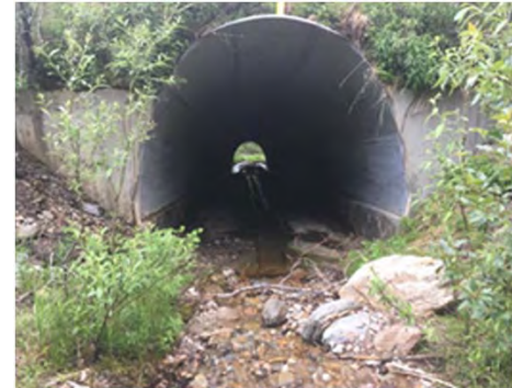
Eagle Creek culvert (~MP 242)
