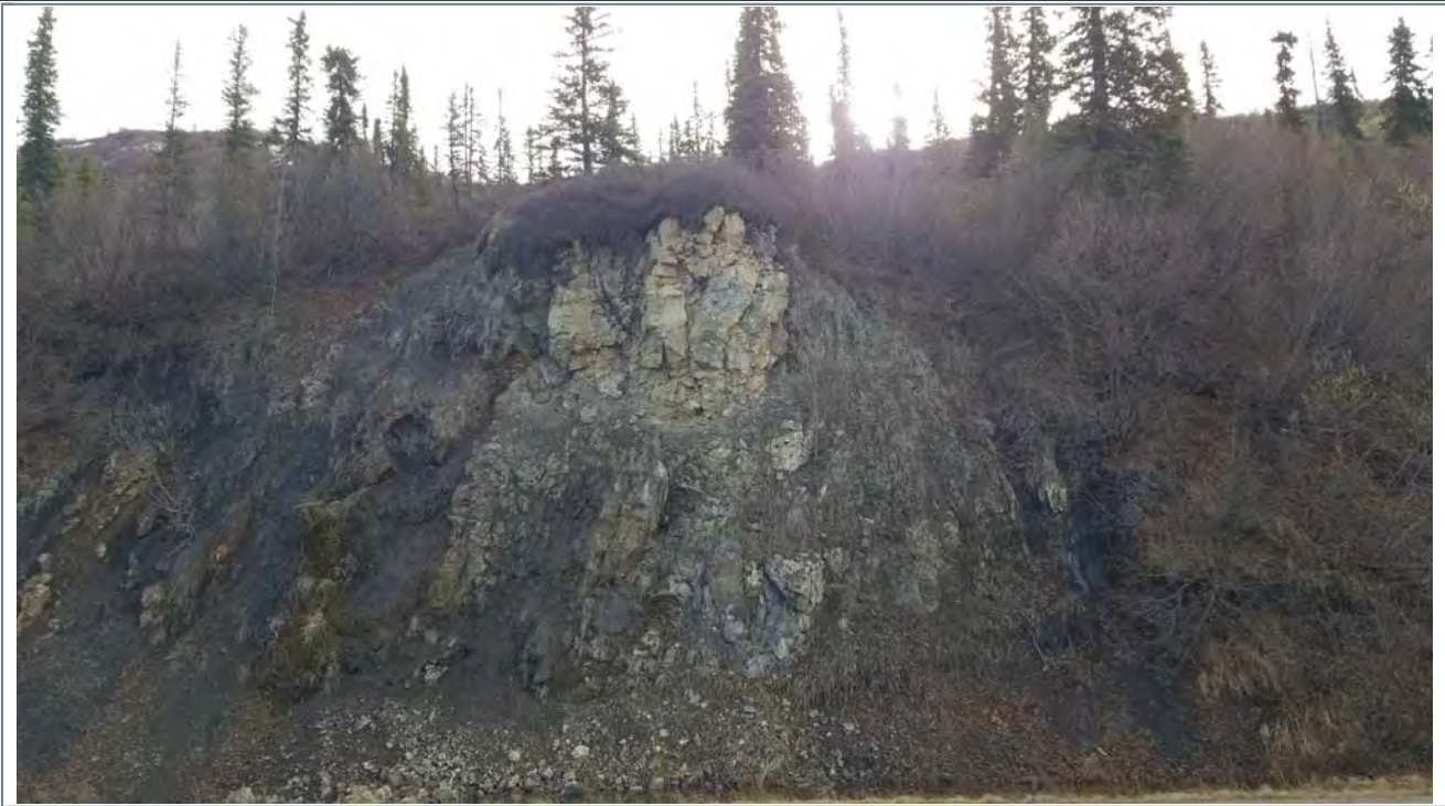
Photo 5: MP 212.3 Potential rockfall hazard.
