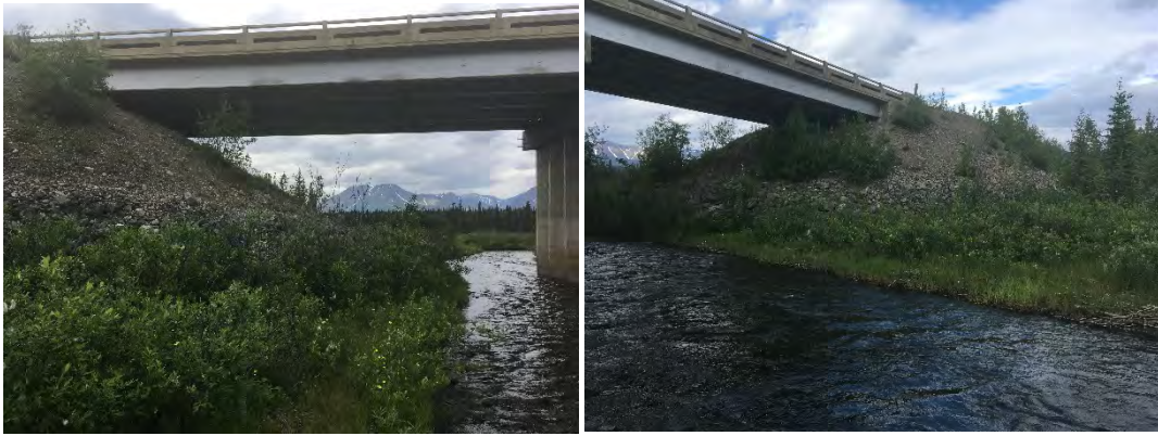
Figure 3. Looking Upstream, Left and Right Abutments
