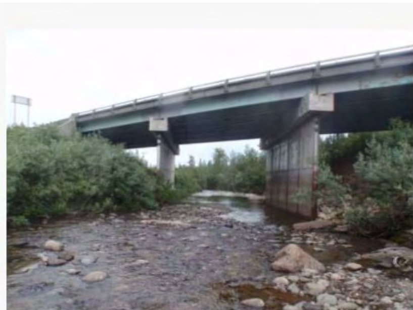
Panguingue Creek Bridge
