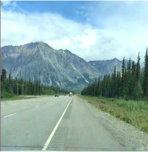
Non-motorized facility solution #2: widened shoulder
