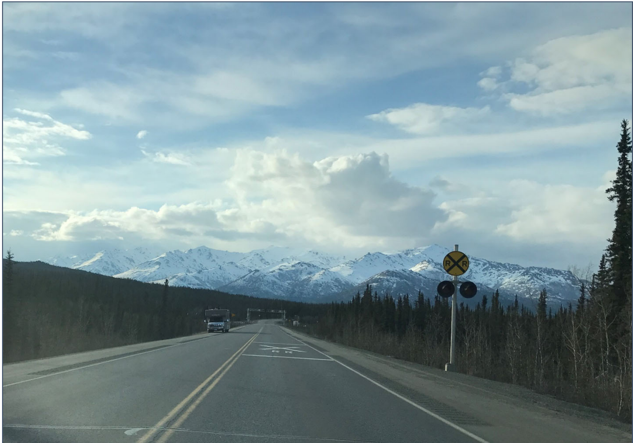
Image of at-grade crossing at Parks Highway MP 235/ ARRC MP 345, looking northbound.
