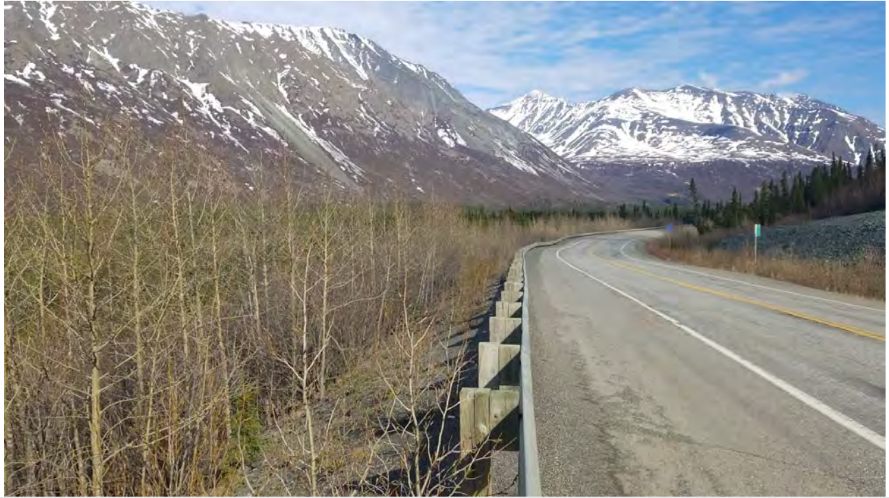
Photo 7: MP 217 Waviness and patching in the roadway. Large dip at MP 217. (SW2020)
