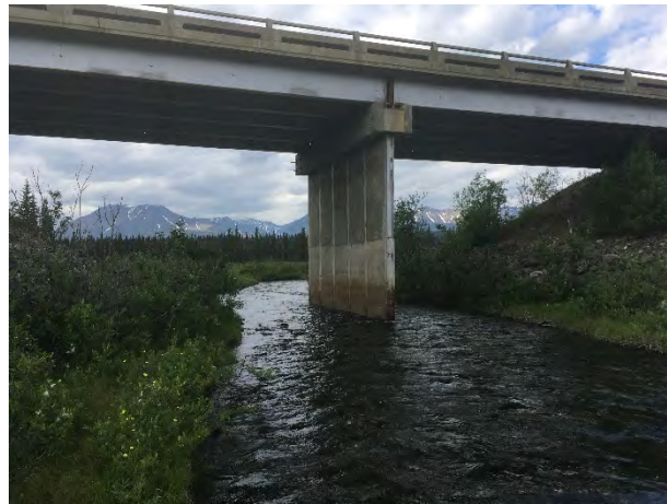
Figure 2. Pass Creek Bridge (BR 0293) Upstream Looking Downstream
