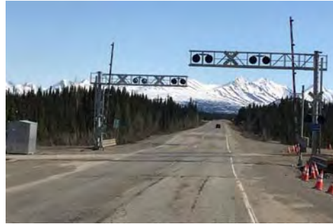
Alaska Railroad crossing maintenance (MP 235)
