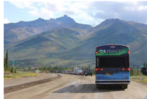
Construction, Tourism (~MP 247)
