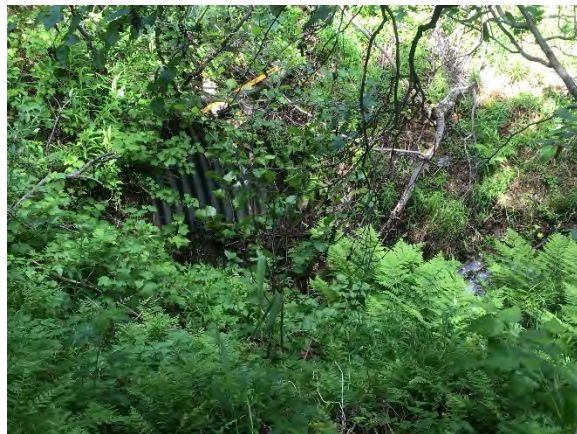
Figure 32. Coyote Creek Cross Culvert, Upstream Side Looking North
