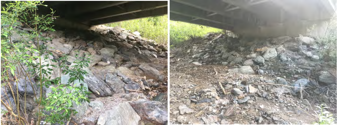
Figure 31. Looking Upstream, Left and Right Abutment
