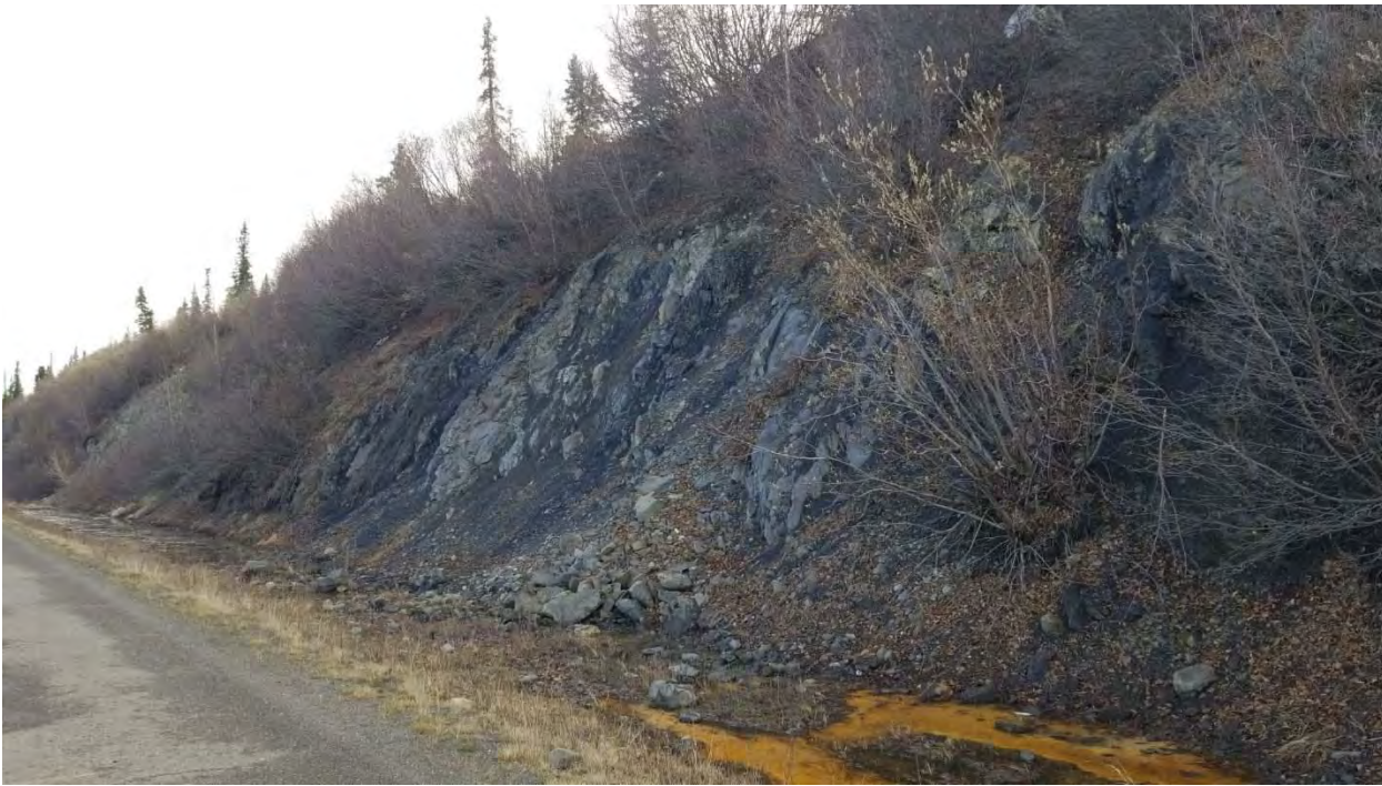
Rockfall near MP 212
