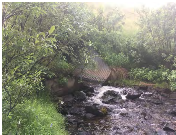
Figure 44. Little Panguingue Creek Cross Culvert, Downstream Looking Upstream
