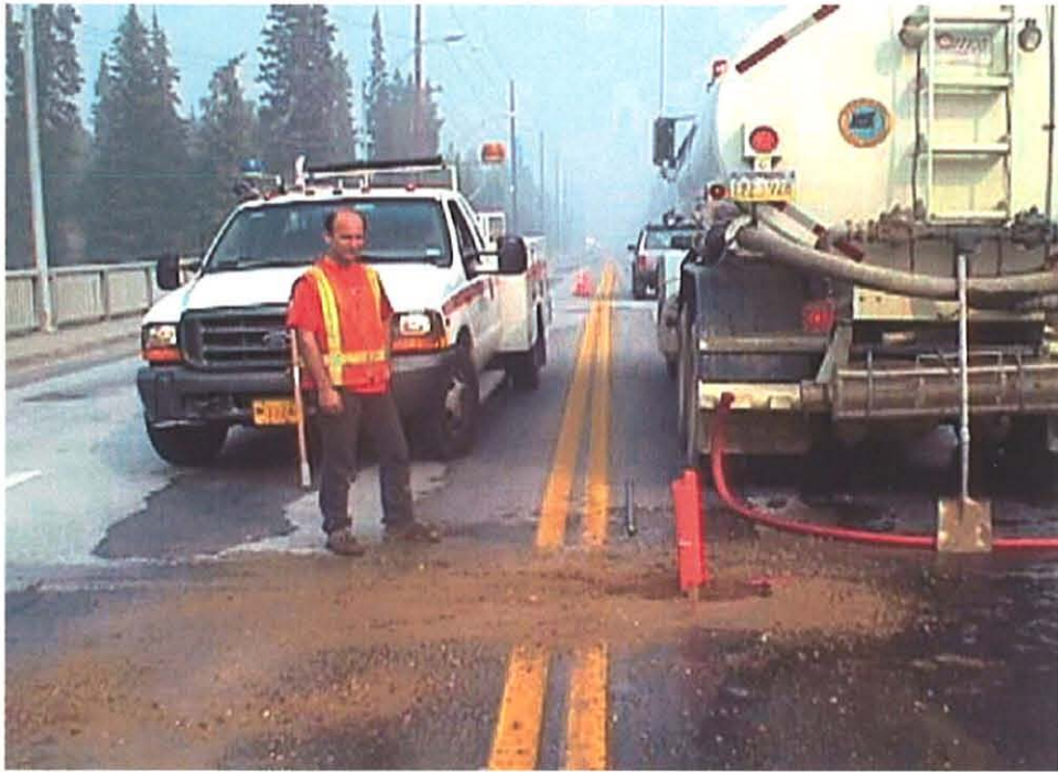
Figure 1.2.4.2 Patching of University Avenue Bridge - August 2004
