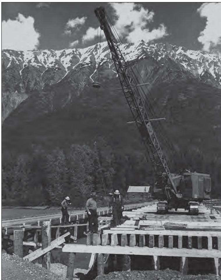
Figure H-8. Erecting the 1943 timber trestle. Sheldon Museum
