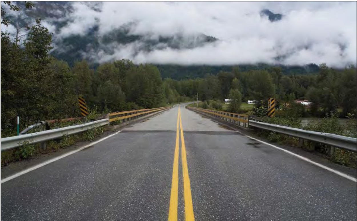
Figure H-11. Approach to the bridge looking southward toward Haines.
