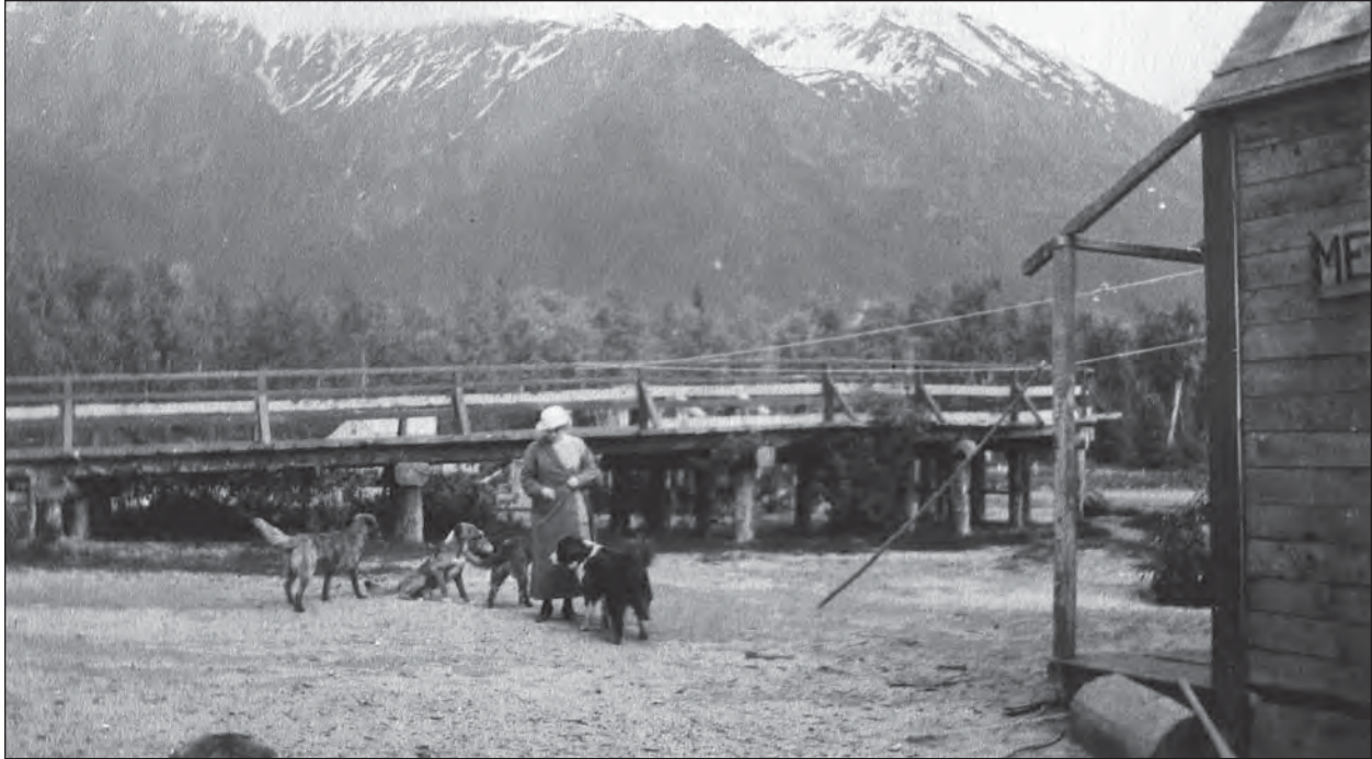
Figure H-4. Northern end of the first Wells trestle showing the curve at the northern bank of the river.
