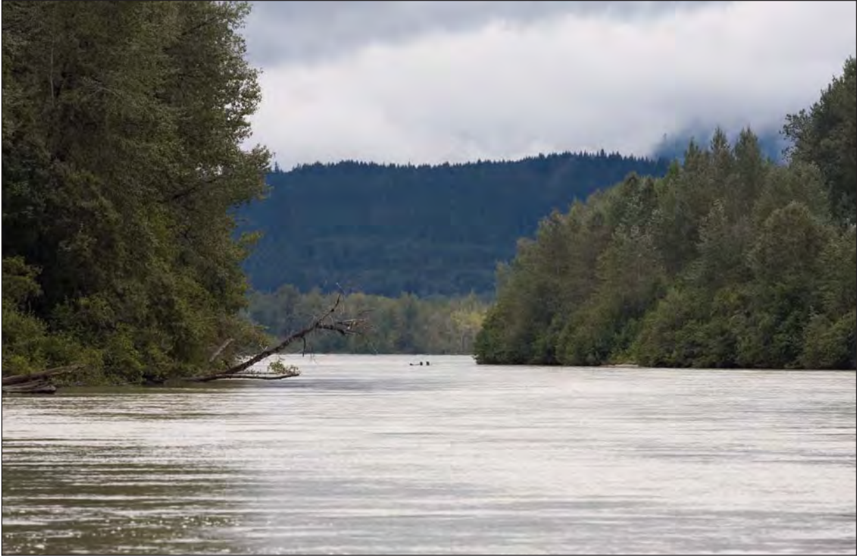
Figure H-2. Old piles in the Chilkat River marking the former location of Dalton Trail trestle (SKG-547), downstream from the current bridge.
