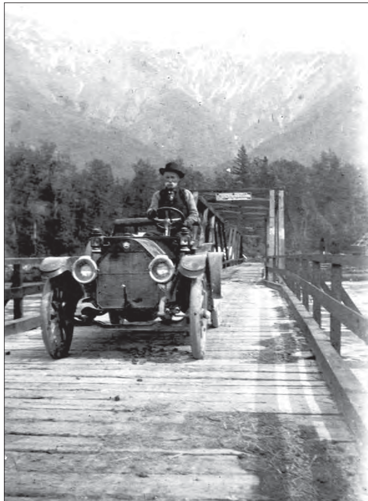
Figure H-6. Vehicle on the first Wells Bridge showing the through truss Howe spans.
