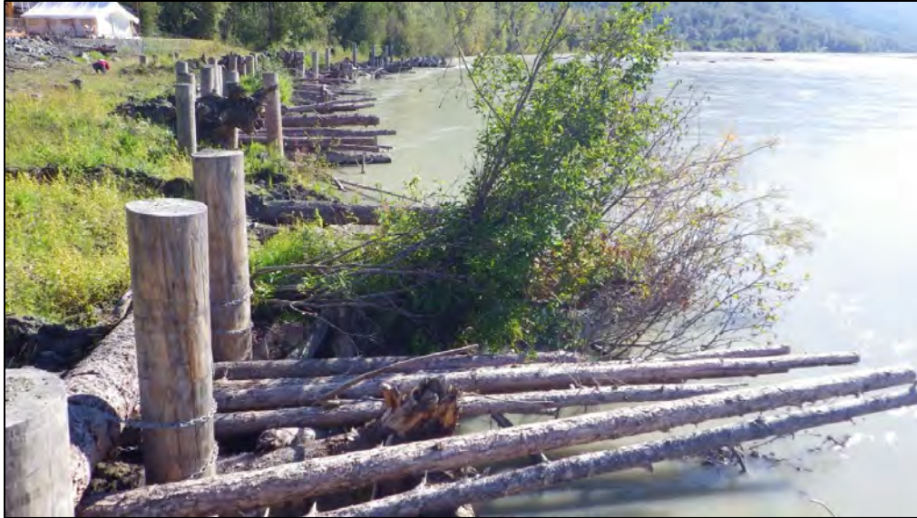
Figure 5. Klukwan wood revetment, looking downstream. (Courtesy ADF&G, 2013).
