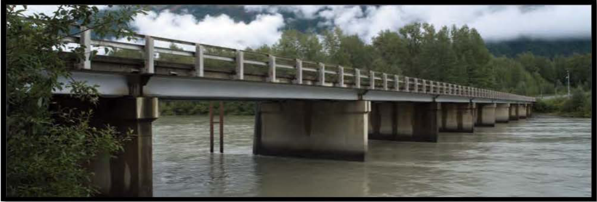
Photograph 1: Chilkat River Bridge
