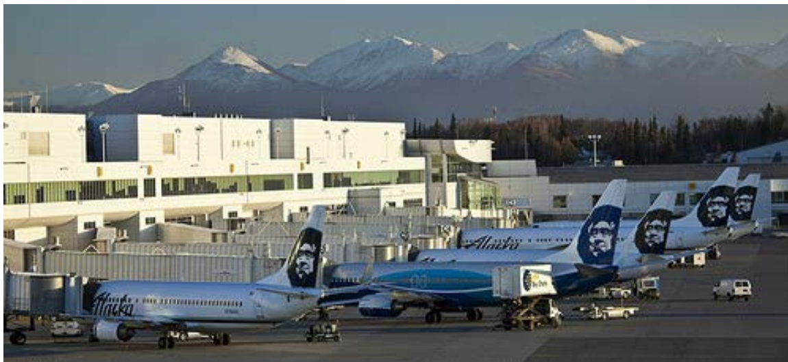
Exhibit 15. Terminal and jetways
