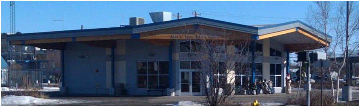
Exhibit 23. Max C. Lyon, Jr. Transit Center in Fairbanks
