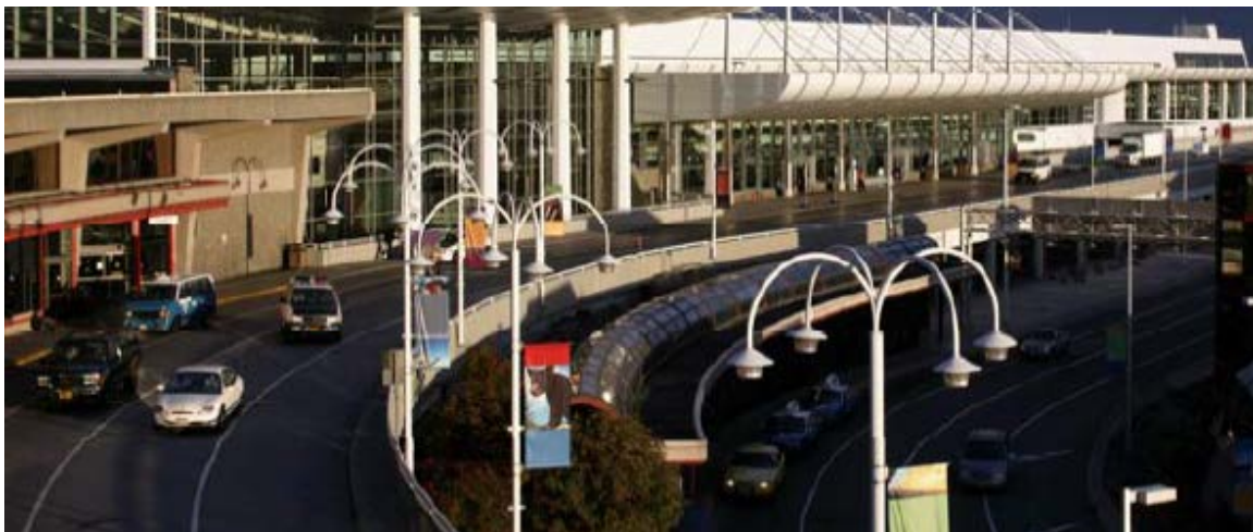
Exhibit 12. Bridge on airport property at ANC
