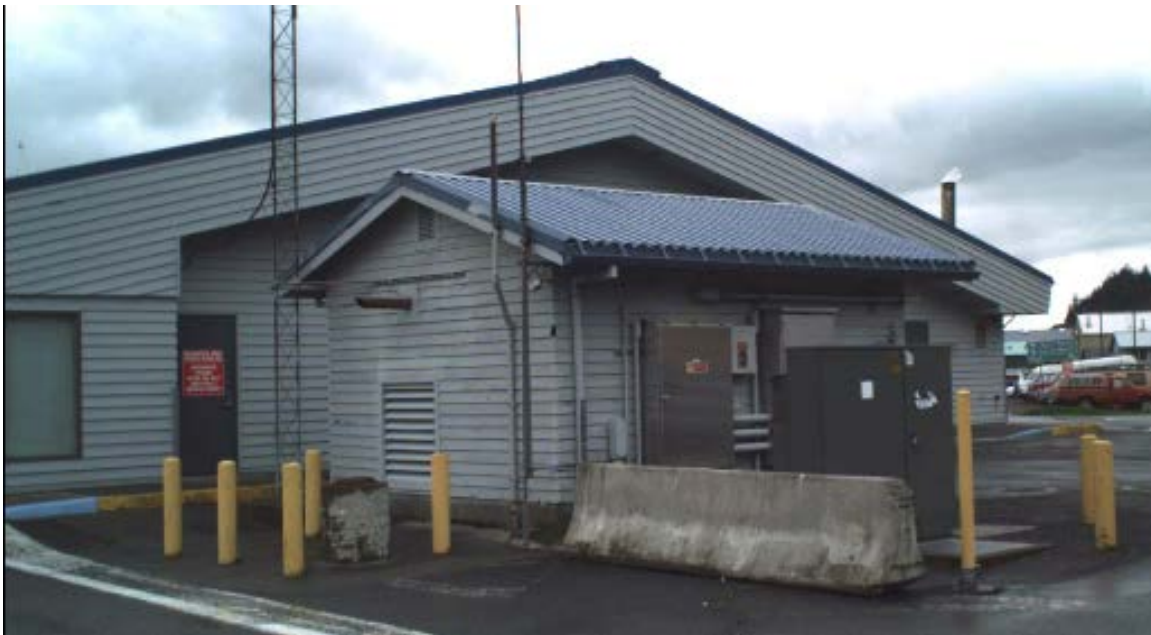
Exhibit 19. Utility building and Ketchikan Ferry Terminal building
